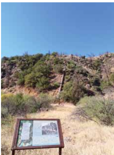
Sally May Siphon Intake
